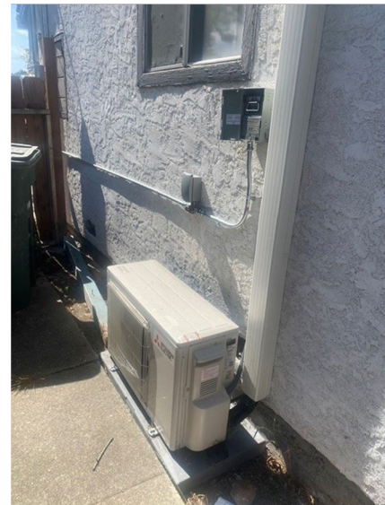
Figure 1: Typical Retrofit Condenser Installation
