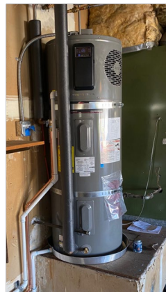
Figure 10: Davis Residence with Upgraded Circuit Splitter and HPWH
