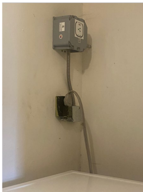
Figure 10: Davis Residence with Upgraded Circuit Splitter and HPWH
