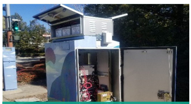
Saratoga Battery Backup at Traffic Light Signals
