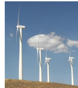
Renewable energy is produced onto the grid
